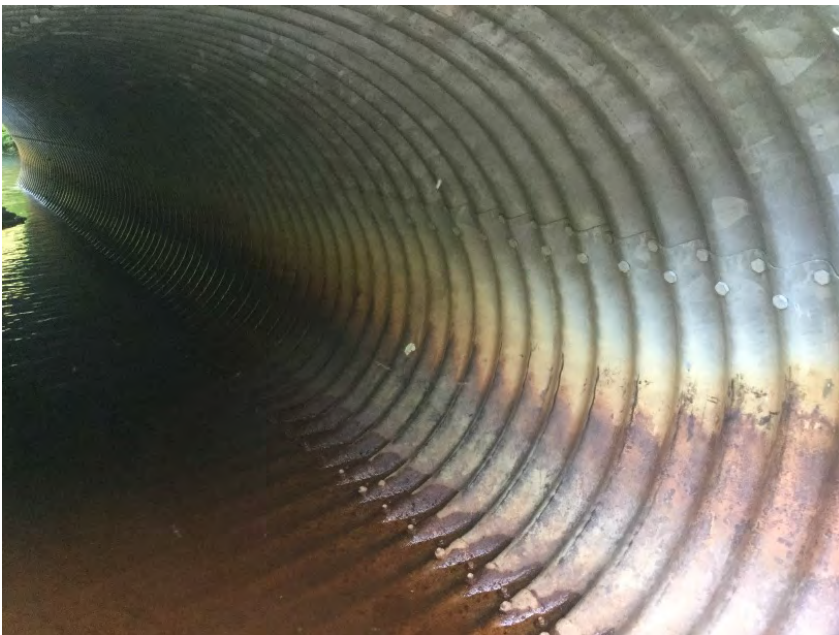
Culvert Barrel Condition
