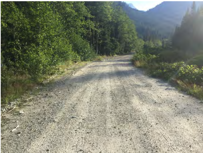
Left Approach Facing Culvert
