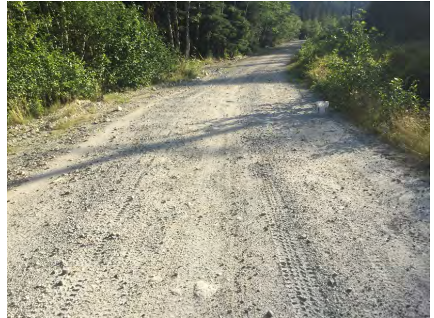
Roadway Over Culvert
