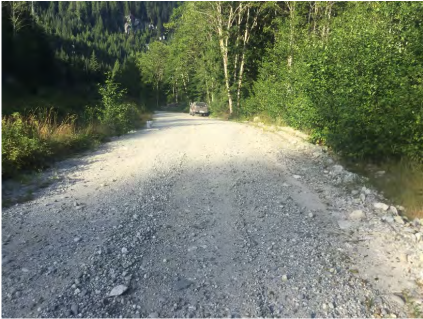
Right Approach Facing Culvert
