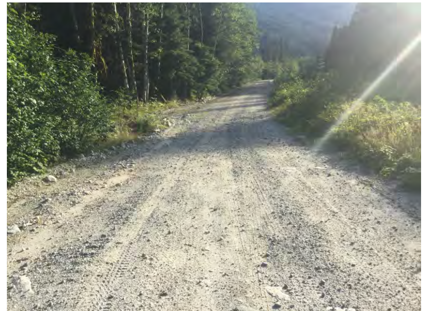
Right Approach Facing Away from Culvert
